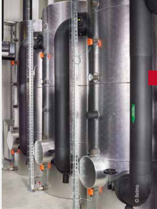
Cold accumulator for optimising the chiller running time.
